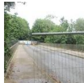
Closure fencing onto the bridge cut and removed
