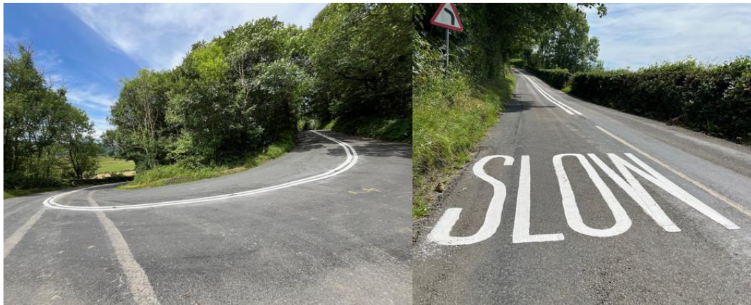
New centre lines and SLOW markings to reduce speed on the diversion route
